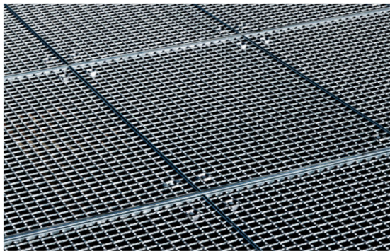
Open grating floor
