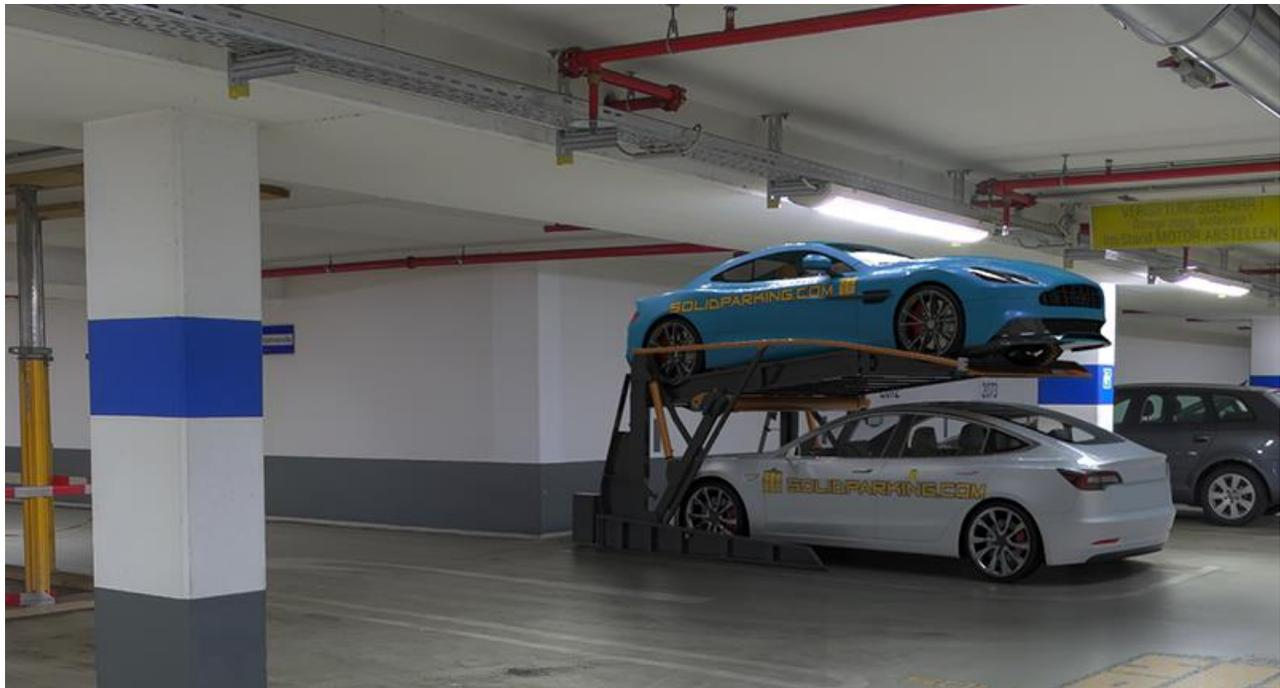
Figure 4. Example of a two-tier car stacker. Source: solidparking.com
