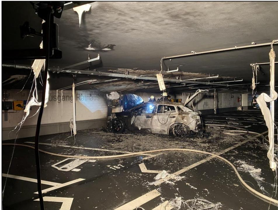
Figure 26. Marienplatz parking garage originating vehicle and surrounding fire scene. (Source: Feuerwehr Ravensburg)
