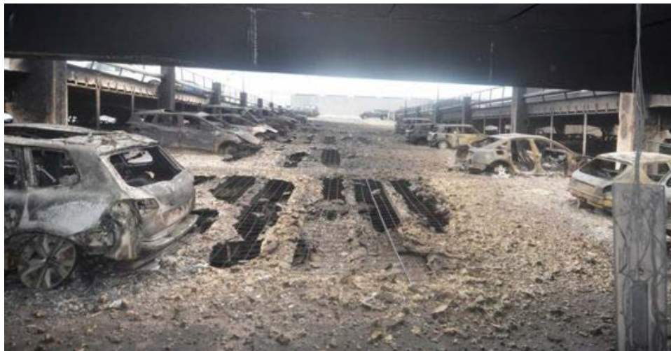
Figure 14 – Concrete spalling in Liverpool, England 2017 fire.
