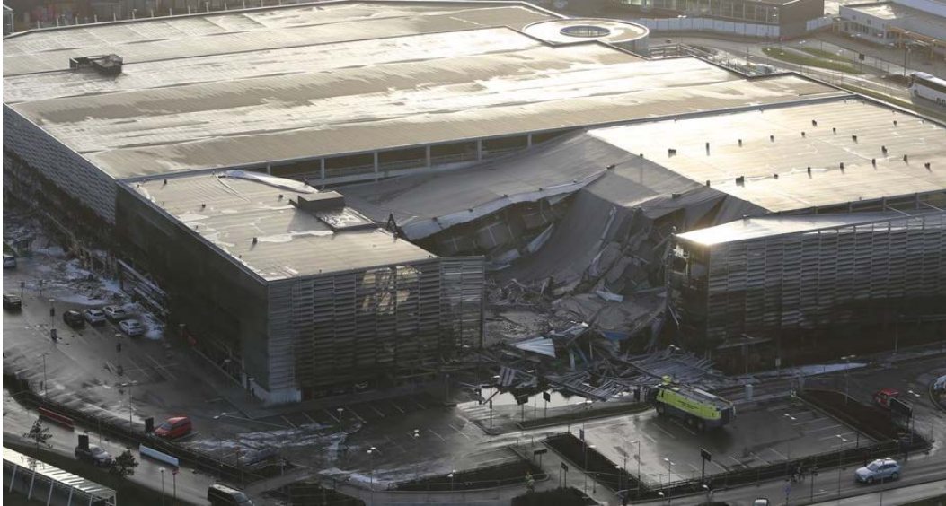
Figure 1 – Partially collapsed parking garage at Norway’s Stavanger Airport after fire in January, 2020.
