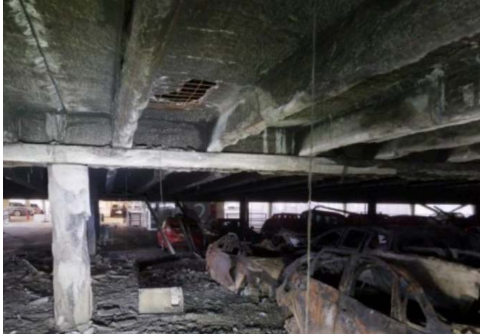
Figure 15 – Concrete spalling in Stavanger, Norway 2020 fire.
