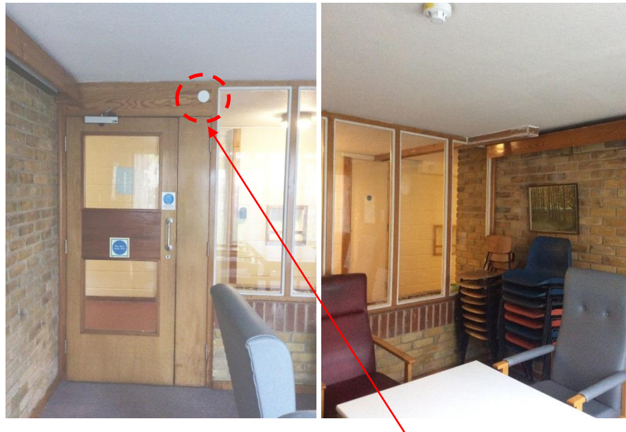
Figure 2 – Photos from Waverley Court. Left image showing the location of the concealed sprinkler head
