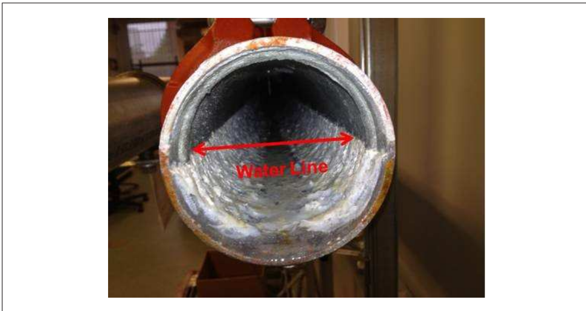
Fig. 4a. Galvanized steel pipe half-filled with tap water in house air after nearly six weeks' exposure
